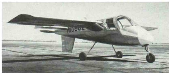
The all-aluminum airplane is light in weight and stands exposure to weather best of all.
